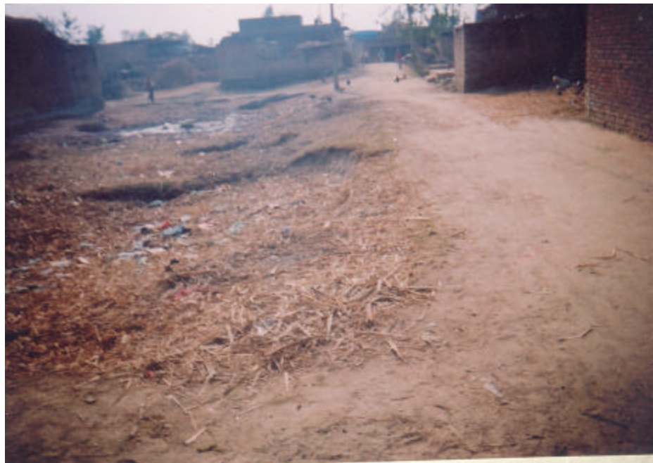
Condition of the Village Roads (Picture - 4)
