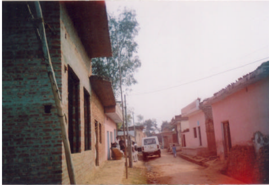
Bamboo Poles for Electricity (Picture - 3)
