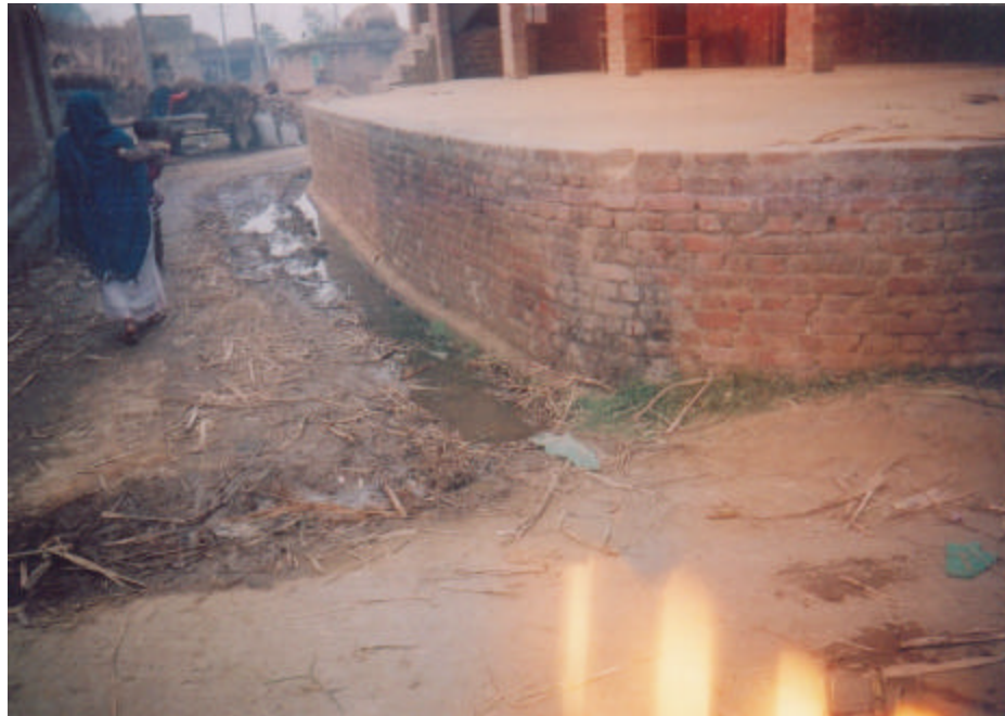
Condition of Drainage System in Village (Picture - 5)
