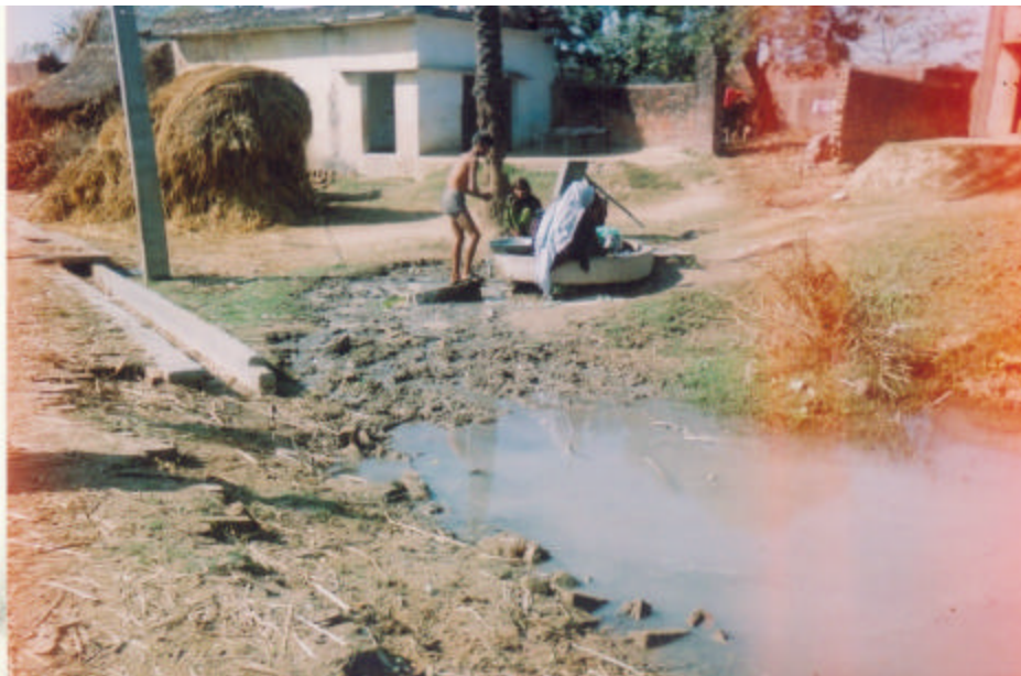
Poor Maintenance of surrounding areas of Hand Pump (Picture - 6)
